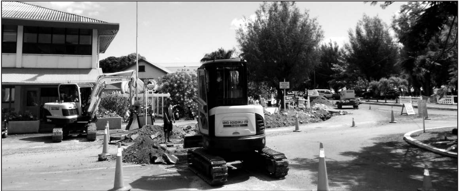
Trenching of sub mains outside court house in Avarua now complete ready for ANZAC Day ceremonies.
